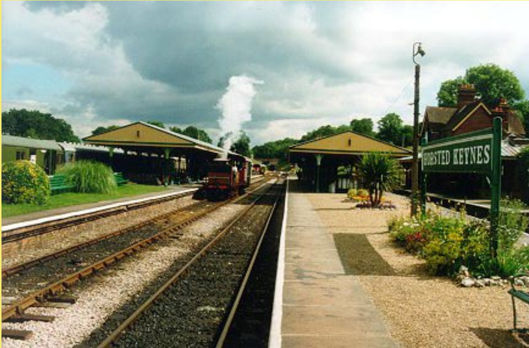
One of the Bluebell's real glories, the expansive Horsted Keynes Station, showing the completed Phase 1 of the Platform 1/2 canopy replacement project. (Richard Salmon)
